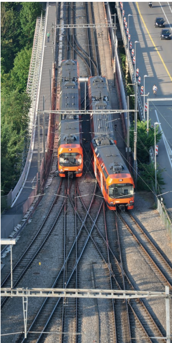
Operations and rail power control linked together.
