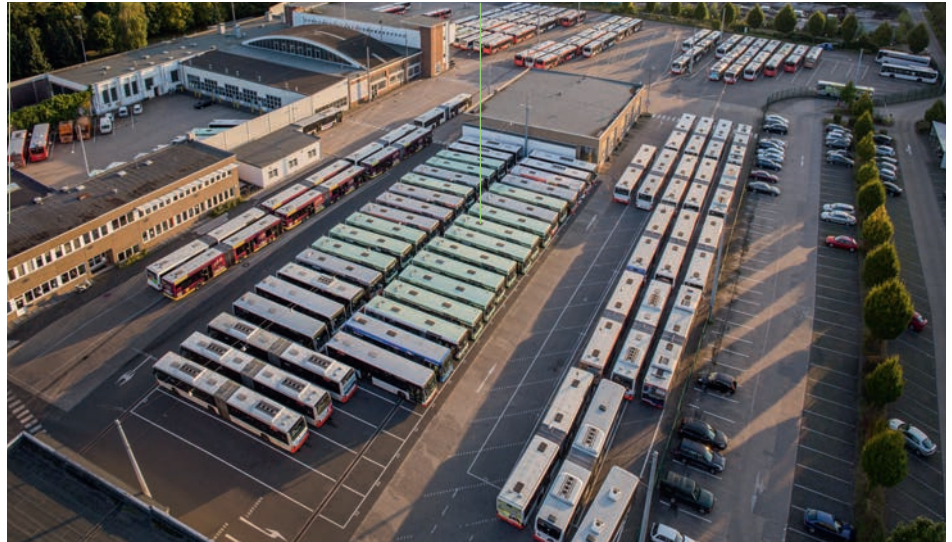
Stadtwerke Bonn, depot in Friesdorf.
