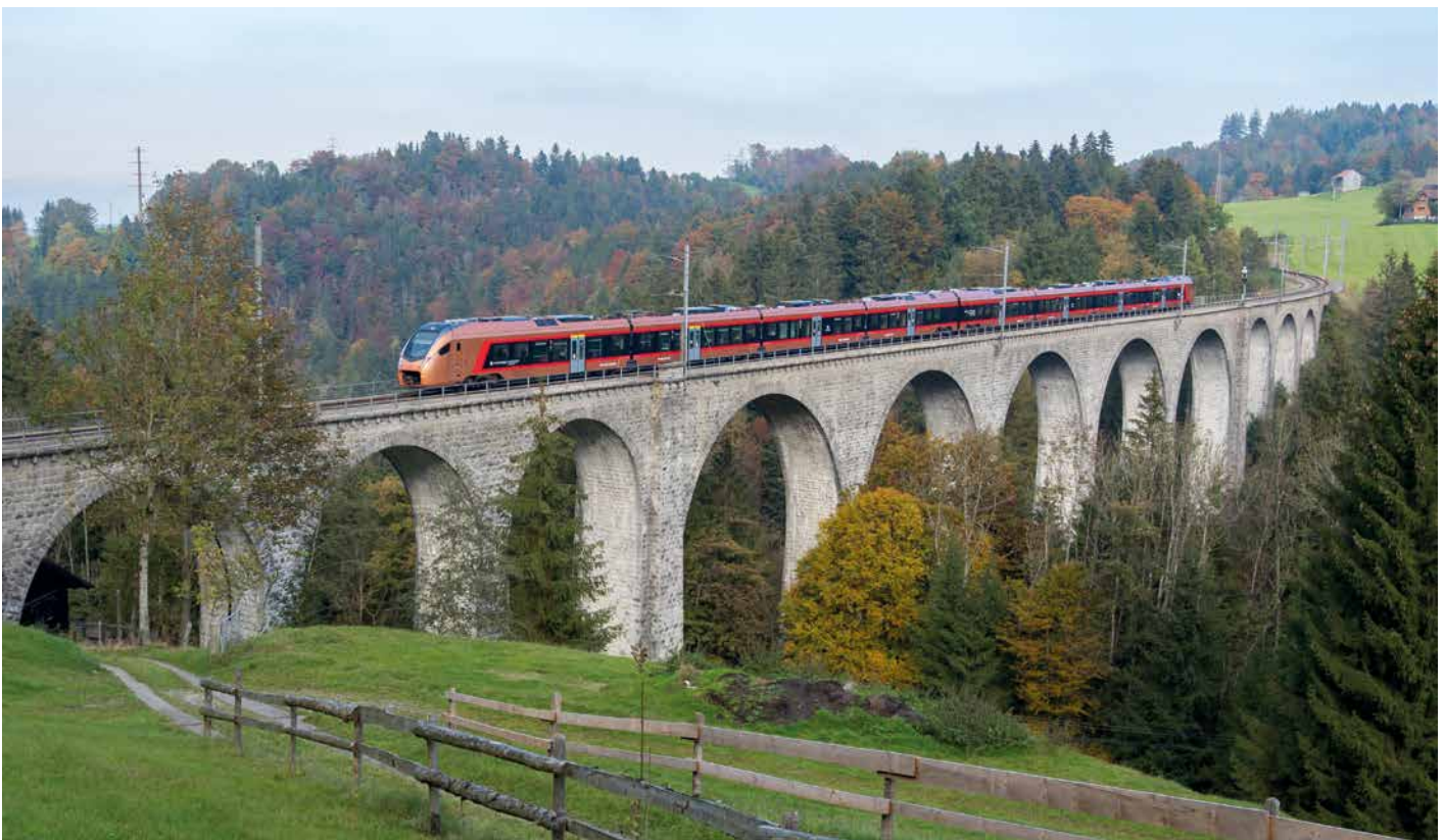
SOB train passes over the Weissenbach viaduct in eastern Switzerland.
