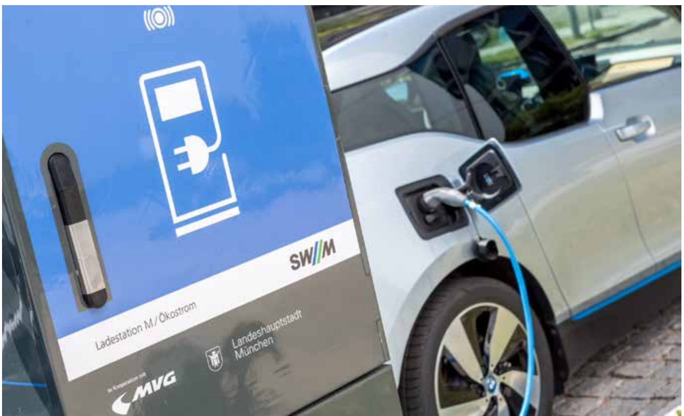
E-charging station of SWM in Munich.
